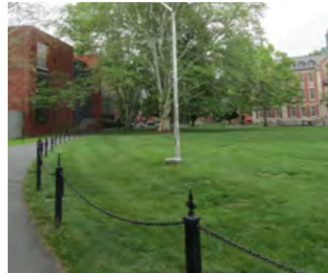
POST AND CHAIN FENCE
