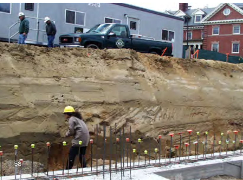
→Soil Profile exposed by construction. Photo by John Brady.
