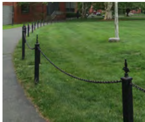
POST AND CHAIN FENCE
