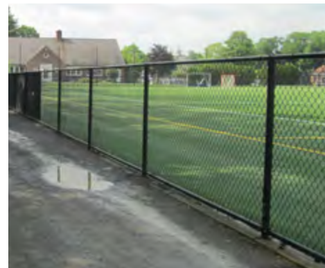
CHAIN LINK FENCE
